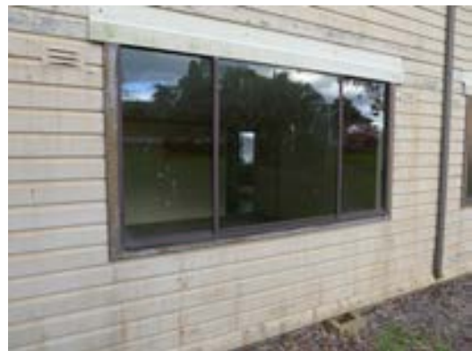
Figure 3. 6: Later addition aluminium framed windows
